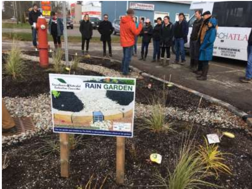
Photo 3: The KWRC rain garden in Sussex helps to store stormwater and filter it slowly back into the ground.
